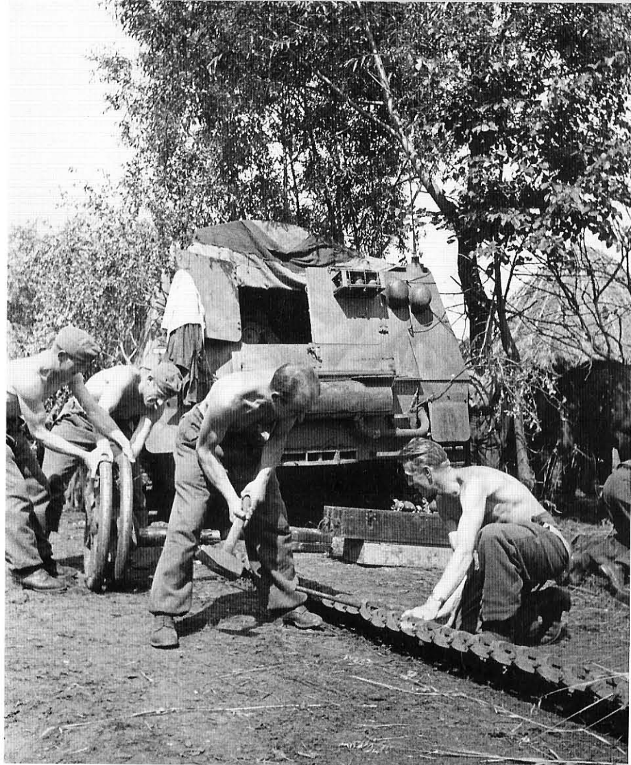
Russia, 1943. Note the dust, mounted vegetation, and mottled field-applied camouflage. Each vehicle crew was trained in the basic maintenance of their vehicle, and here replace the track pins with the tools carried in the fighting compartment.
