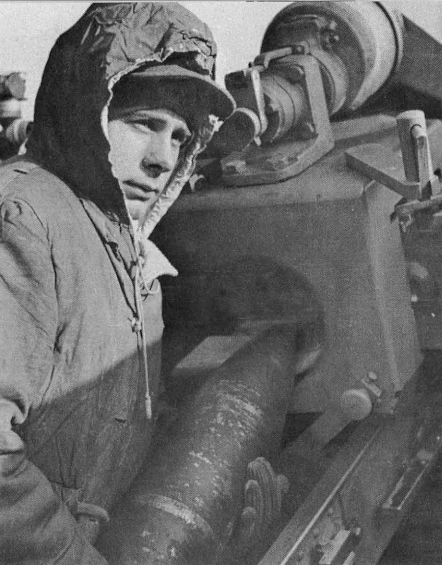
The loader stands before the opened breech of the 15 cm howitzer with a 96 pound high explosive projectile in his hands. The handle that opens and closes the horizontally sliding breech is visible on the right hand side of the breechblock.
